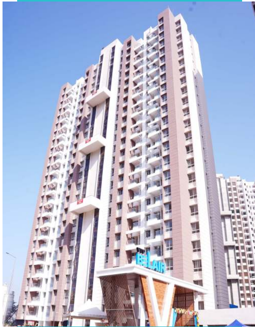
VTP BEL AIR 1, 2 & 3 bedroom homes, Mahalunge
